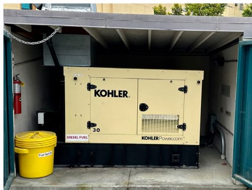
Fire Station 93 Emergency Generator Replacement Project. The new emergency generator replaces one that was 36-years old. The typical estimated useful life (EUL) of an emergency generator is 20-years.
