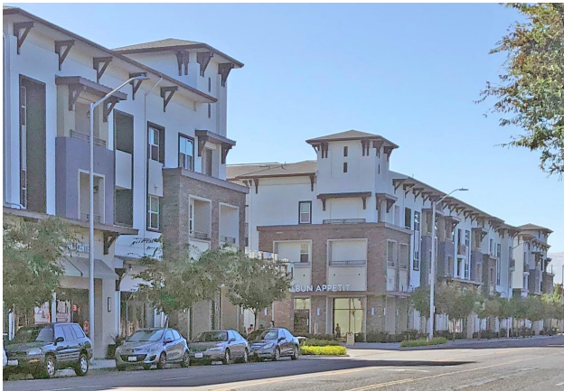
Embedded corner tower element for a mixed-use building.
