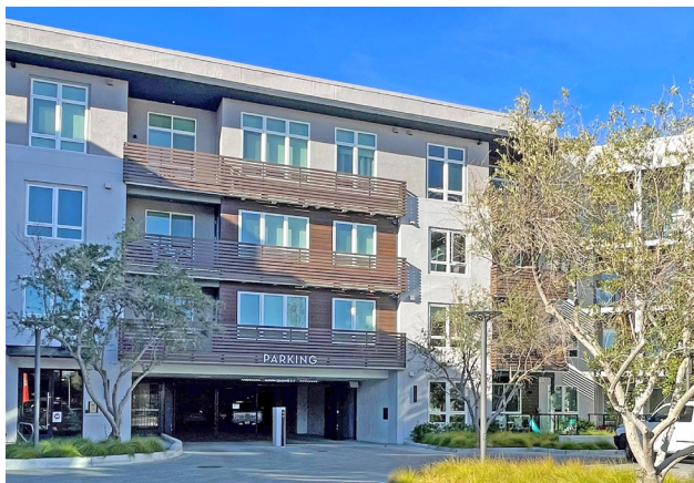
Multifamily residential project with podium parking on the ground floor.
