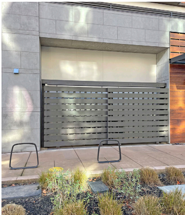
Trash collection area screened from public view by a metal gate of durable material.
