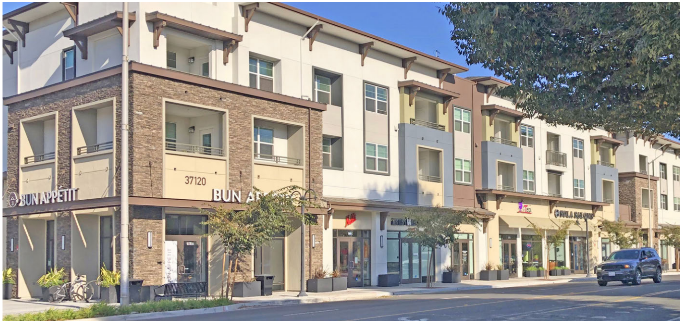
Mixed-use development with building entrances facing primary street and with ground floor height of at least 12 feet.
