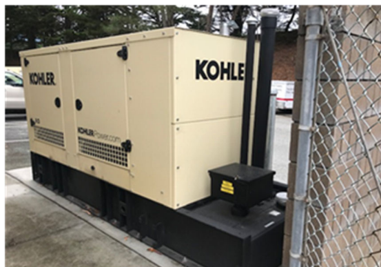
Fire Station 94 Generator Replacement Project: Stand-by generators have an estimated useful life of twenty years. The new generator replaced a 48-year-old generator that powered half of the facility. The new generator provides emergency power to the entire facility.
