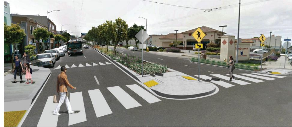
The Mission Street Streetscape Project will improve pedestrian safety and beautify Mission Street between Crocker and Templeton Avenue. The project will widen the existing concrete median from 3 to 7 feet, plant drought-tolerant median landscaping and install an irrigation system.
