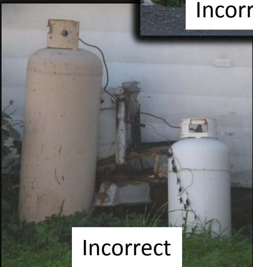
LP-gas vessels are not secured to prevent accidental over turning. Provide an approved method to secure and support LP-gas containers and vessels. (e.g. secured to the unit's hitch, a support post, or other approved means) [25CCR 1208, 1211]
