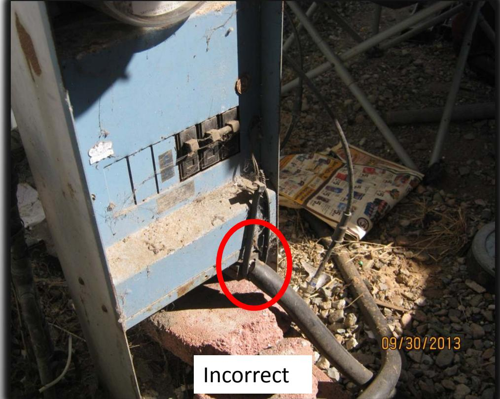
The power cord covering is cracked or deteriorated exposing the conductors. Replace the cord with a cord listed for manufactured home/mobilehome or recreational vehicle use, as appropriate. [25 CCR 1352(a)(1), 1606(d), 1607(d)]
