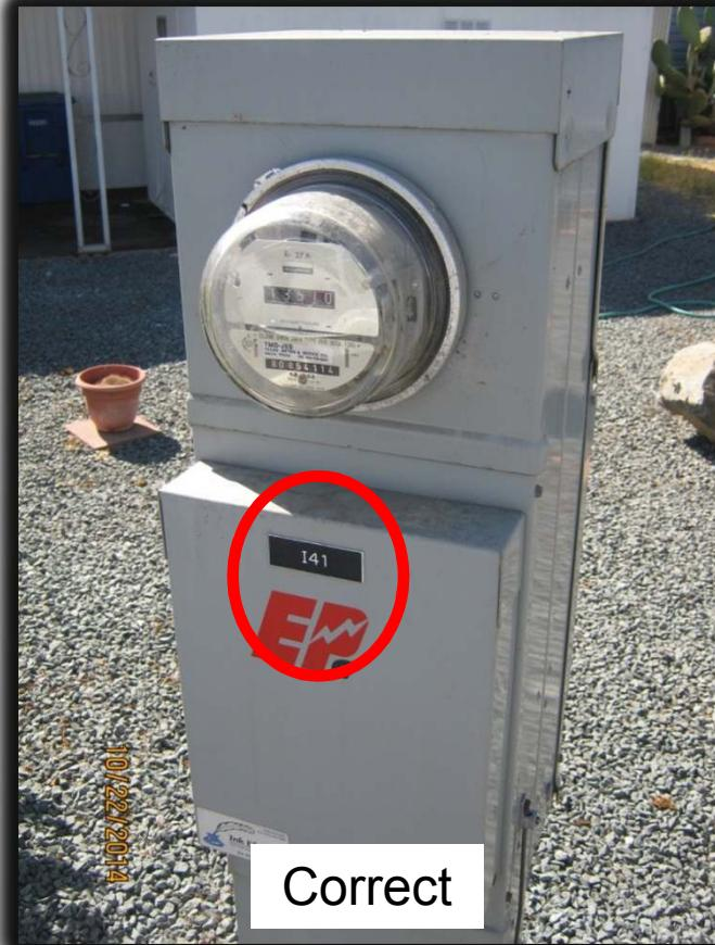
The electrical distribution panels, overcurrent devices, fuses or switches which serve the space, fixture, device or other equipment controlled at the distribution panels are not clearly and permanently marked. Clearly and permanently mark electrical distribution panels, overcurrent device, fuses or switches to identify the space, fixture, device or other equipment controlled at each distribution panel. [25 CCR 1134(a), 1151; Reference: California Electrical Code, Article 110-22, 230-70]
