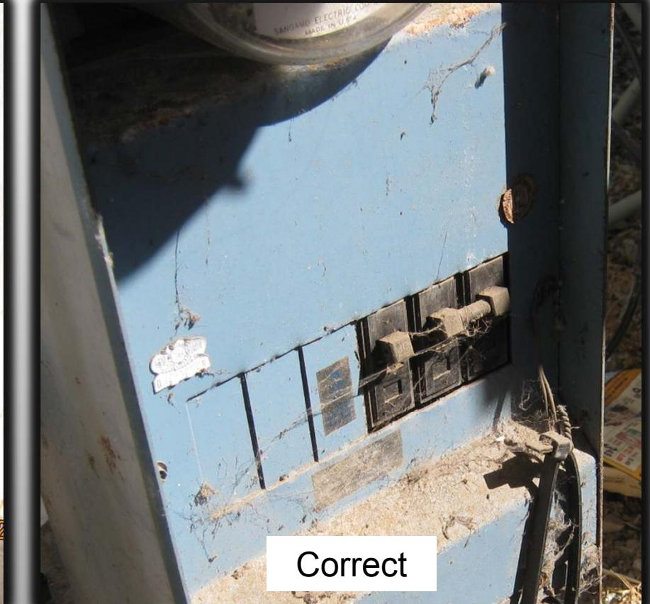
The lot/park electrical service equipment has exposed or easily accessible live electrical parts. Cover all exposed live electrical parts and plug unused openings in electrical equipment. [25 CCR 1134(a), 1188(b); Reference: California Electrical Code, Article. 230-62]
