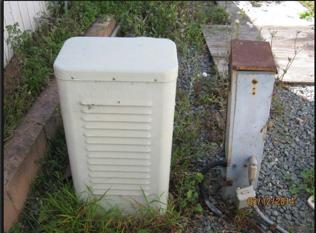
The park/lot electrical service equipment is not accessible for inspection, repair, or disconnection in case of emergency. Provide unobstructed working clearance of at least 30 inches wide by 30 inches deep and 78 high in front of the electrical equipment. [25 CCR 1183; Reference: California Electrical Code, Article 110-26]
