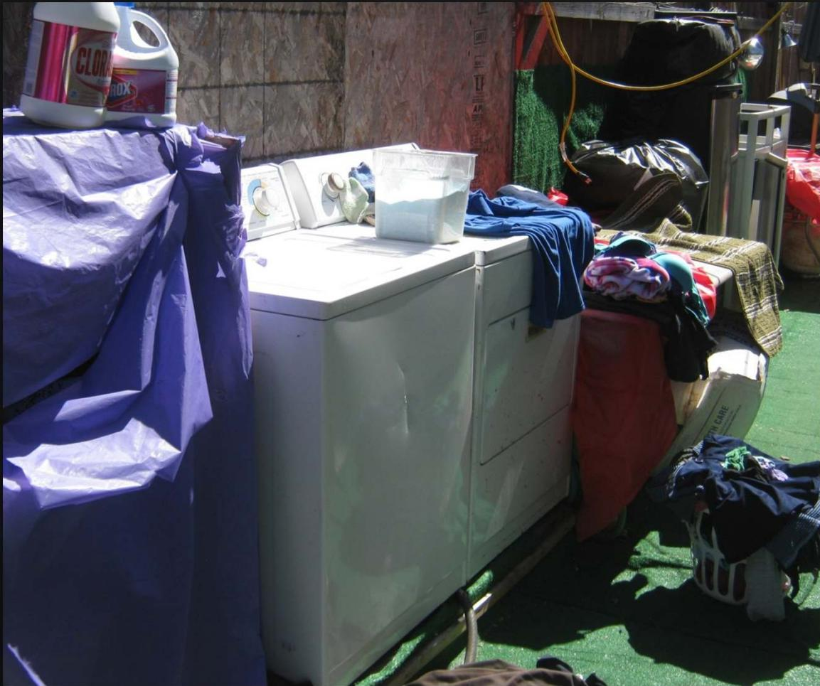
Appliances shall not be installed outside of the unit exposed to the weather or connected with an extension cord. Relocate the appliance(s) out of the weather and/or remove the extension cord. [25 CCR 1134(a), 1188(b), (d)]
