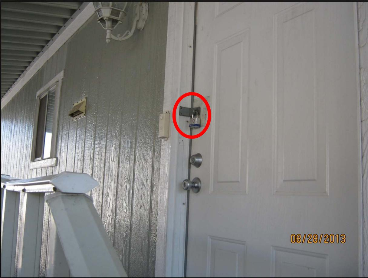
One or more required exterior egress doors are blocked or locked with an exterior hasp, preventing emergency exit. Remove the material or hasp from in front of the doors and provide for proper exiting. [25 1606(c), 1607(c), 1608(c)]
