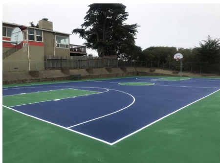
Tennis & Basketball Court Surface Rehabilitation Project: Base failure repair and acrylic resurfacing of approximately 64,430 square feet of sport courts. The existing worn out basketball systems were replaced at Gellert Park, Lincoln Park, and Palisades Park.
