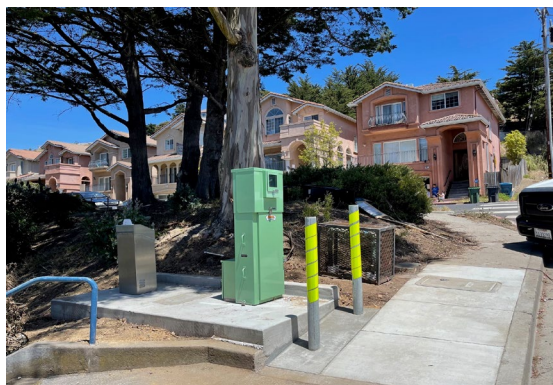
Edgewood Park Electrical Service Panel Replacement: Electrical service cabinets of this type have an estimated useful life of 20-year. The new electrical service cabinet replaces one that was over 40-years old.
