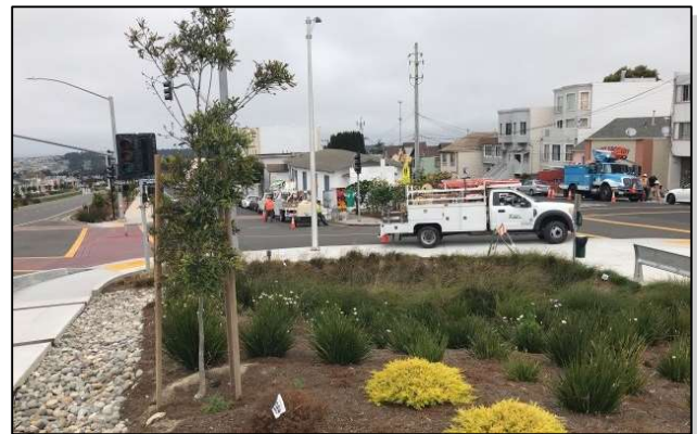
Example of a green infrastructure project: landscaped medians and bioswales on John Daly Boulevard.
