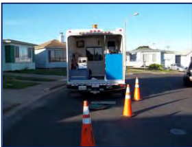
Traffic Control Setup
