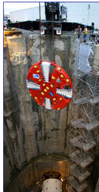
Figure 5-7 Typical construction shaft
