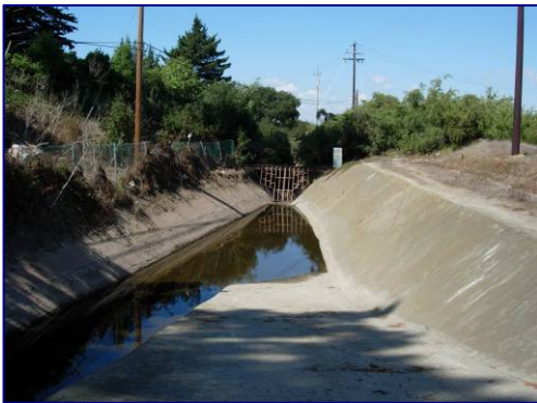
Figure ES-4 Vista Grande Tunnel Entrance
