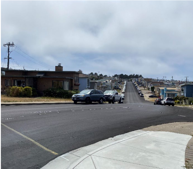
Ocean Grove Avenue: Skyline Slurry Seal provides pavement preservation for roads in the Skyline neighborhood of Daly City.
