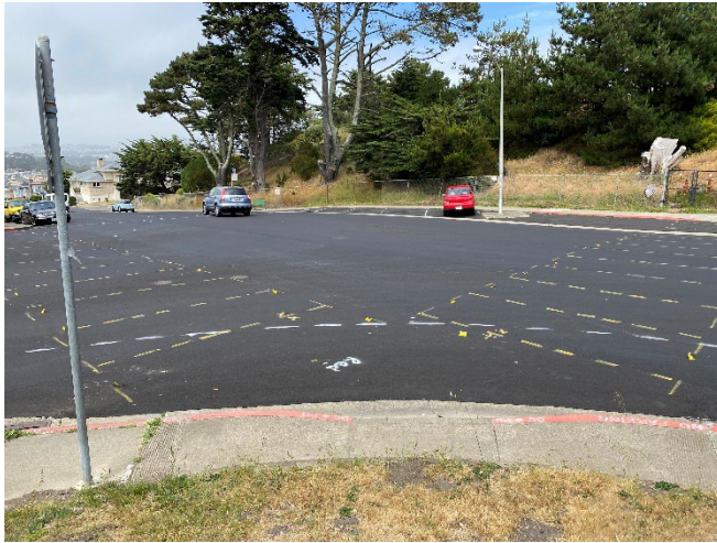
Westridge Avenue: Westmoor Avenue and Westridge Avenue Intersections Quick Build project received grant funds to install painted bulb-outs and high-visibility crosswalks to increase pedestrian visibility along two corridors identified on the City's High Injury Network.
