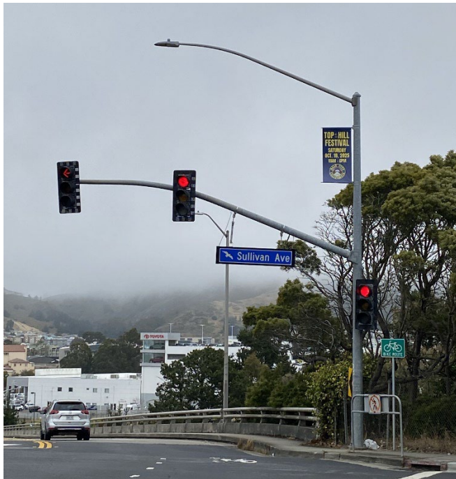
Sullivan Avenue/San Pedro Road: Replacement of old internally illuminated street name signs throughout the City with energy efficient LED street name signs.
