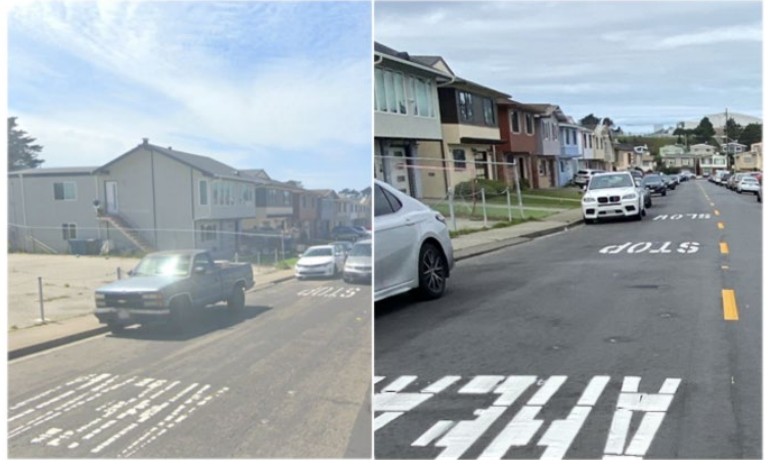
San Fernando Way: 2022-23 Street Resurfacing Project included pavement base failure report and asphalt concrete overlay for several streets for a pavement useful life of 15 years.
