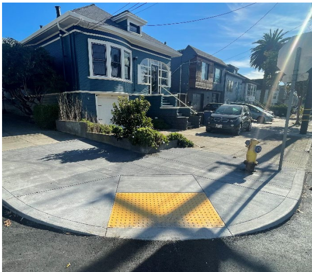
Vista Grande Ave & San Diego Ave: ADA/Sidewalk Improvements Project constructed curb ramps and sidewalk improvements.
