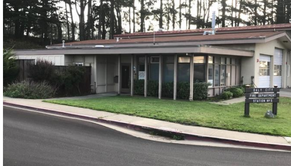
Fire Station 95: The roof of Fire Station 95 was redone to provide a useful life of 50 years.
