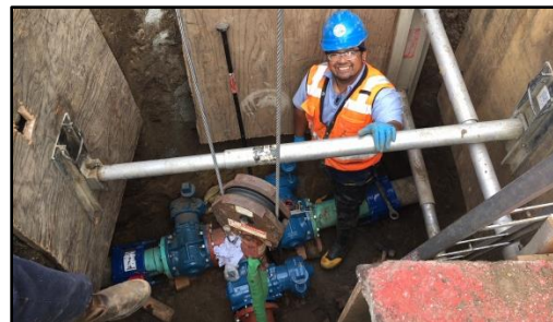
Tie-In Valve Installation
