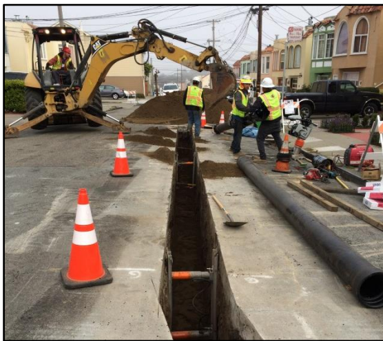
Water main replacement
