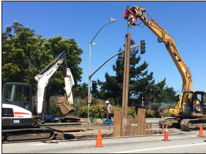
Junipero Serra: Sewer main replacement
