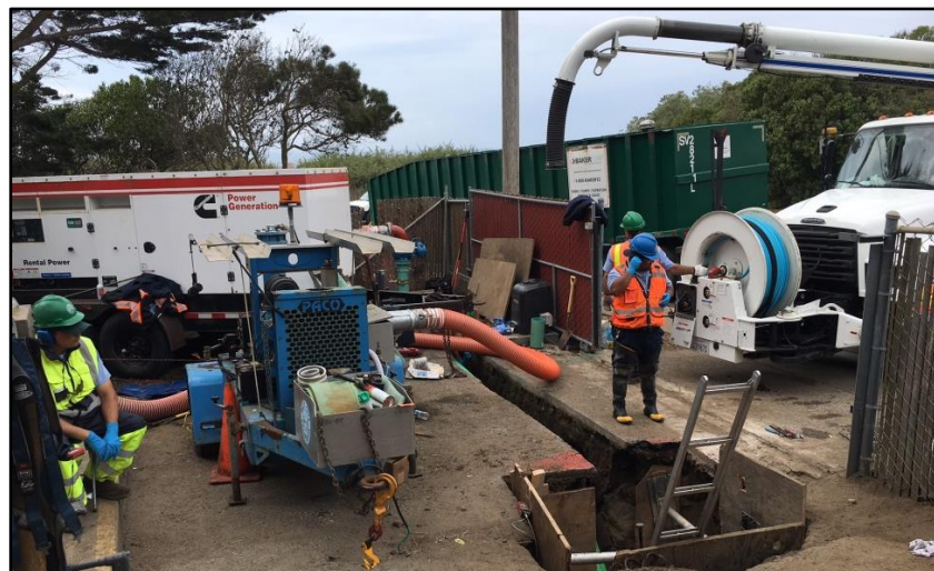
Skyline Lift Station: Emergency Bypass Installation
