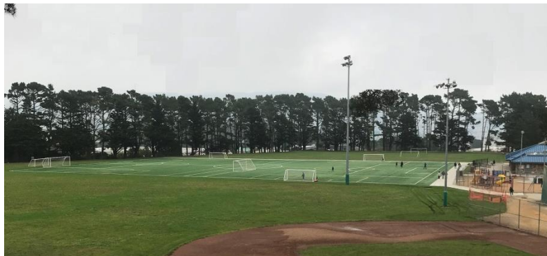
Gellert Park: The outdated artificial turf soccer field was replaced with a safer and more environmentally friendly product.
