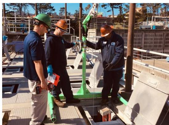
Senior Water/Wastewater Operator, Brandon Wardle, is working with Plant and Equipment Maintenance staff, Charlie Michielsen and Hassan Shah, in clearing a plugged drain line in one of the wastewater treatment plant's tertiary treatment system filter cells. The cell that is being worked on is one of 12 individual, sand filtration cells in the tertiary recycled water process.
