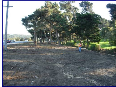
Figure ES-14 Area Along Existing Canal Proposed for Construction of the Vista Grande Wetland
