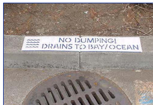
Figure ES-17 Ongoing Nonstructural BMP Implementation in Daly City
