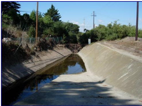
Figure ES-4 Vista Grande Tunnel Entrance
